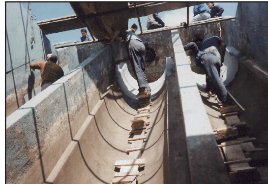
ARC 791 applied to properly prepared surfaces
